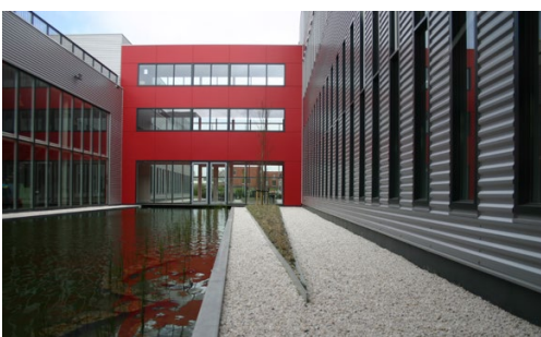
service access route around the building
